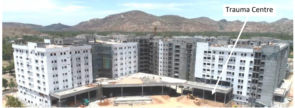
Kannigapuram hospital nearing completion
